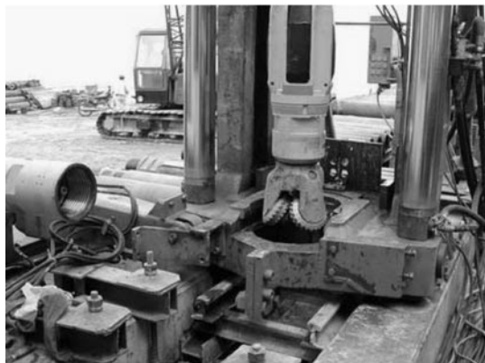
Photo 1. Directional Drilling System for pilot hole drilling, Raise boring method
