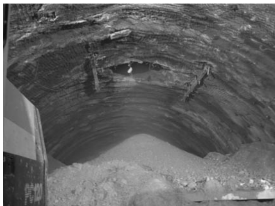
Photo 3. Mucking during reaming operation, raise boring method
