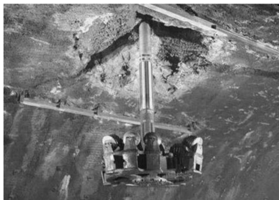
Photo 2. Drill bit for reaming, raise boring construction method
